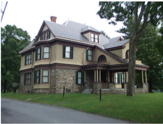
Deyo House today
